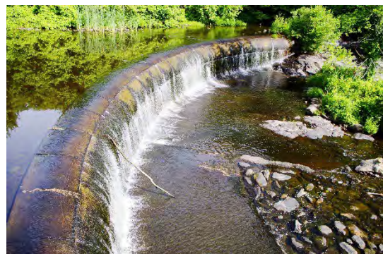
The Quinapoxet Dam concrete arched spillway
