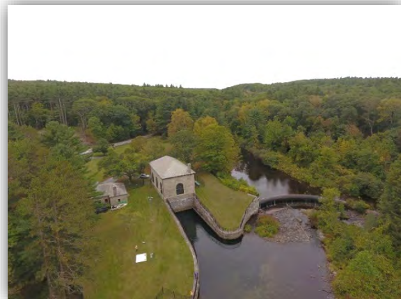
Figure 1: Oakdale/Shaft 1 (L) and Quinapoxet Dam (R)
