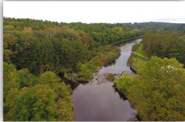
Figure 2: Quinapoxet Dam view from upstream
