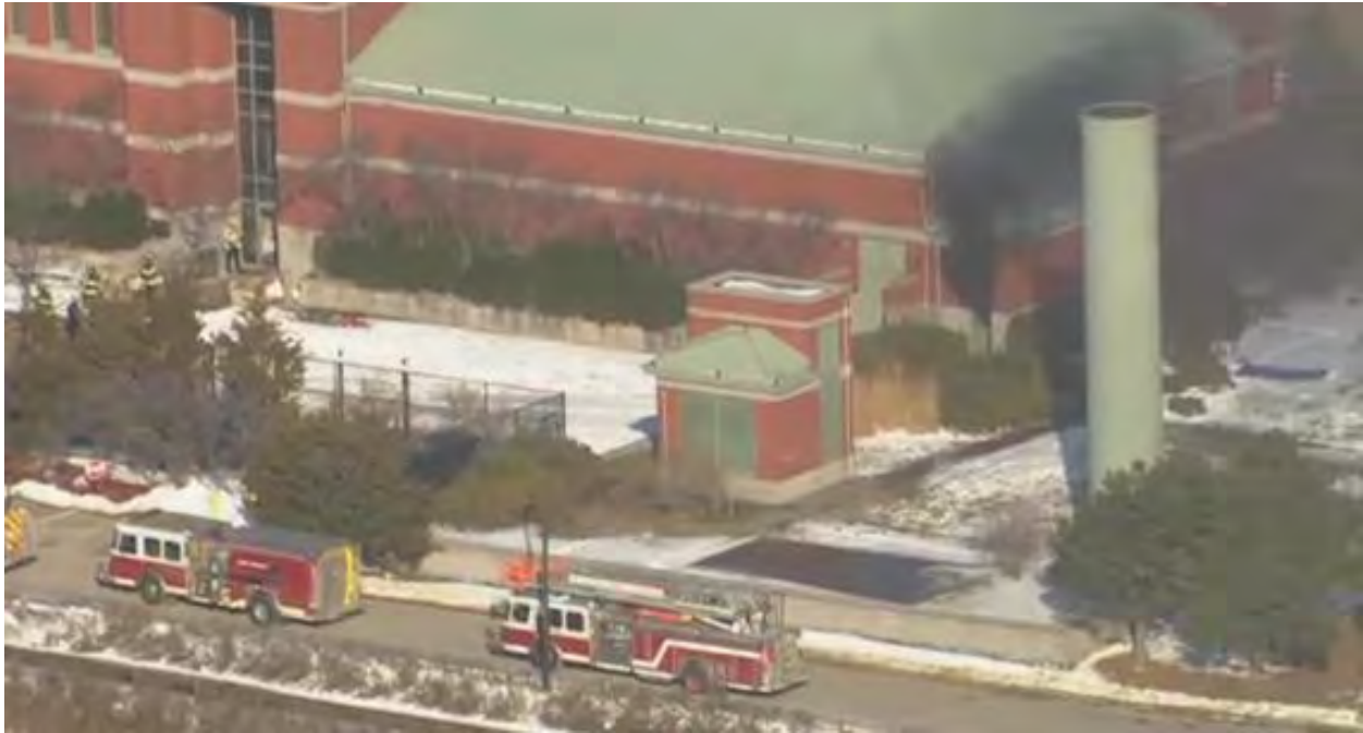
January 2016 Fire in Odor Control Room
