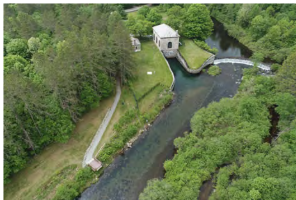
To the right in this photo, the Quinapoxet Dam spans the Quinapoxet River. To the left, MWRA’s Quabbin Aqueduct Shaft 1 Oakdale Power Station and Quabbin Aqueduct Service Building
