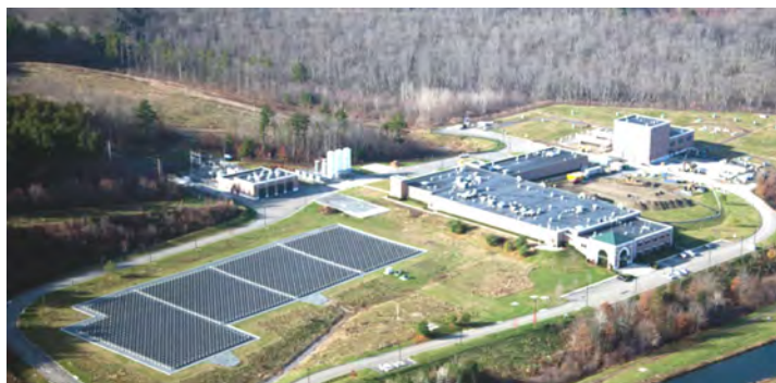
John J. Carroll Water Treatment Plant
