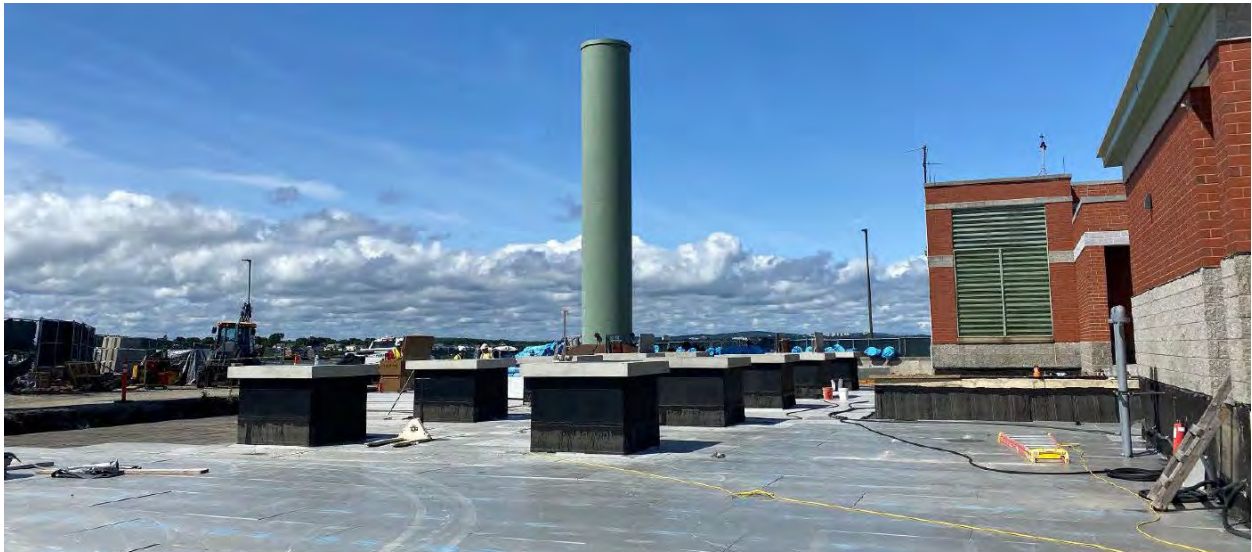
Roof of Odor Control Room Prior to Replacement of Soils
